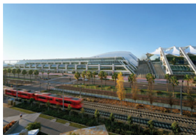
The San Diego Convention Center, home to ACG 2013. Photo courtesy of: Timothy Hursley
